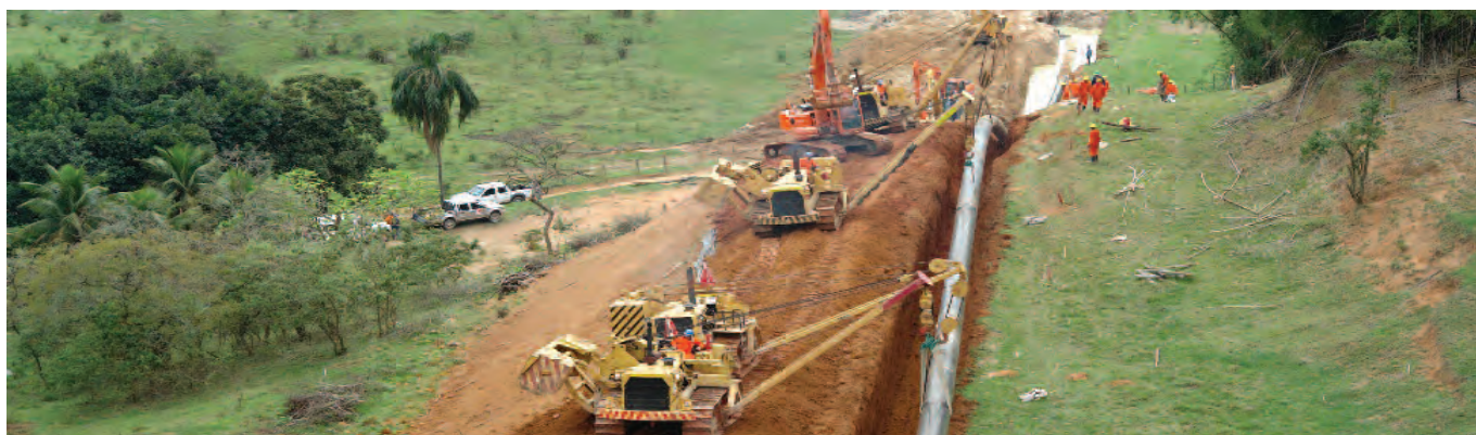
Deployment of pipelines to transport natural gas on a stretch of rising hill, using tube settlers, hydraulic excavators and other heavy equipment.
