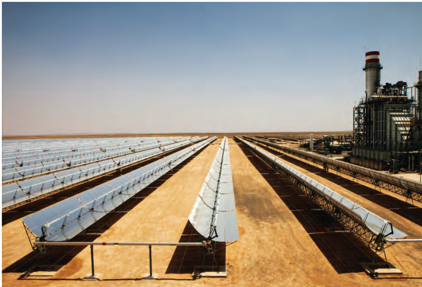
Alternatives to fracking. The Ain Beni Mathar Solar Plant in Morocco. The solar plant is the first hybrid combined solar cycle plant worldwide. It has a 470 MW capacity and avoids 33,000 tonnes CO 2 emissions per year. © Markel Redondo/Greenpeace
